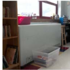
BEL Replace through-wall heating units
