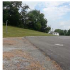
CES Additional Asphalt for parking
