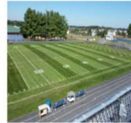
AHS Stadium Bleachers, paved pathways, restroom additions
