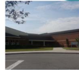
EMHS Weight Room & Locker Room Additions (CIP type project)
