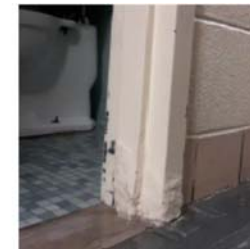
MBE Cut out door jams and weld new pieces
