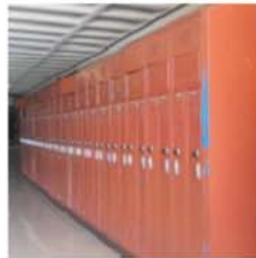
CHS Replace lockers
