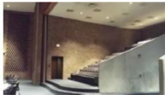
CHS Replace the second Auditorium Moveable Partition
