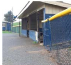
CHS Replace baseball field backstop & add new ticket gate and fence
