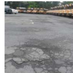
Cambria, Technology, Montgomery Central Pave/overlay asphalt parking lots
