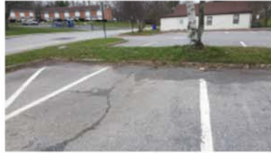
HAE Overlay/re-pave asphalt parking lots and drives, rebuild curbs, Increase number of marked and paved parking spots.
