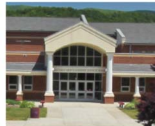
EMHS handicap auto door openers at main entrance
