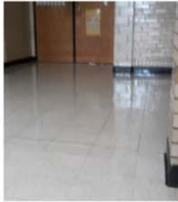
SMS Replace floor tile
