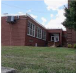
SMS Replace handicap ramp at front
