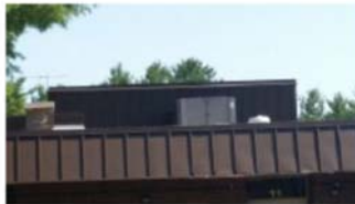
CPS HVAC Unit replacements
