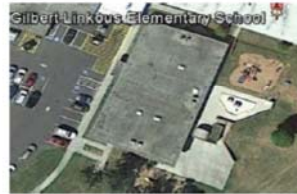
MBE & GLE Kindergarten Buildings HVAC Unit Replacements
