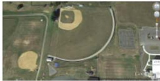
AHS baseball field dugout improvements
