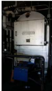
CPS Install new boiler - CT
