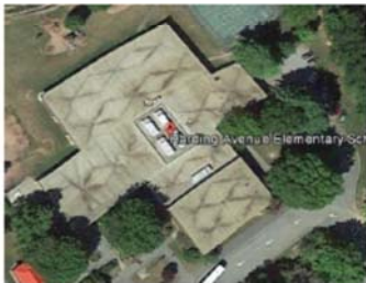
HAE HVAC Units Replacement?
