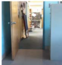
GLE replace office flooring
