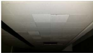
CHS, SMS Replace ceiling tile and ACM abatement (SMS)
