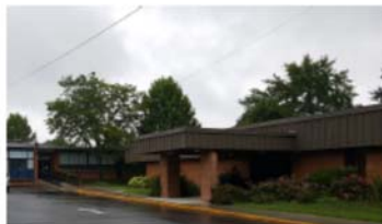
MBE Construct canopy from school to kindergarten
